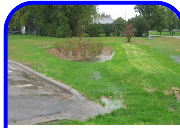
Flows greater than \frac{1}{2} inch water quality volume bypass the cells through overflow weirs set at 9 inches higher than the surface elevation of the bioretention cells.
