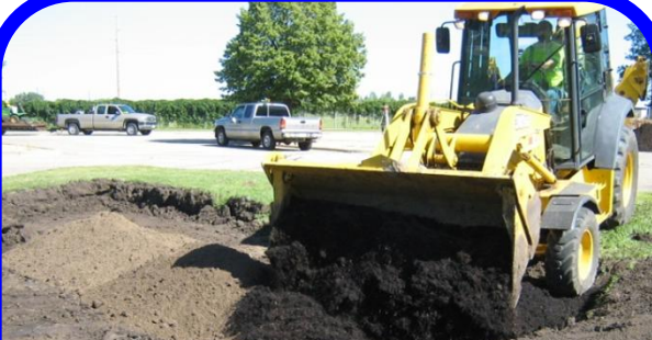
In existing soil was amended with coarse washed sand and leaf litter compost. Mixing to a 12" depth helped to remove soil compaction.
