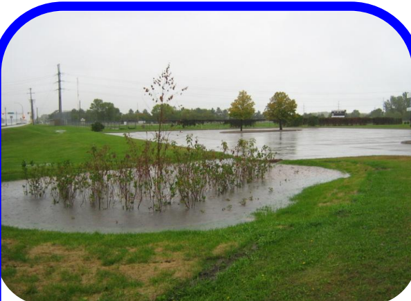
The designed water quality volume of \frac{1}{2} inch runoff depth fills the cells to capacity. The temporary pool infiltrates within 12 hours following the rain event.
