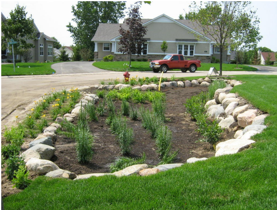
Rainwater Garden Installed at the Pearlmont Heights Development Photo courtesy of Dakota County SWCD
